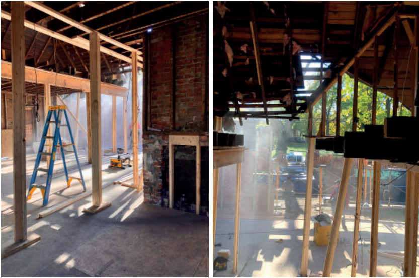
OCT 2020 Demolition, deconstruction, and construction processes overlap with design.
