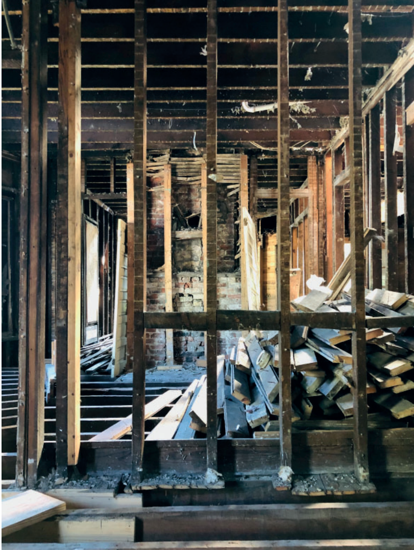
SEPT 2020 Recovering material to repair and replace or reposition during demolition and deconstruction.
