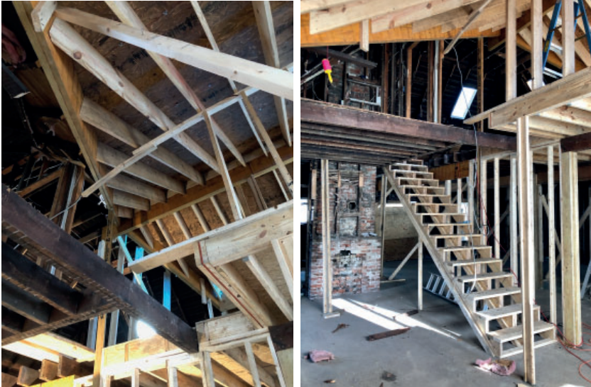
WINTER 2021 Demolition, deconstruction, and construction processes overlap with design.
