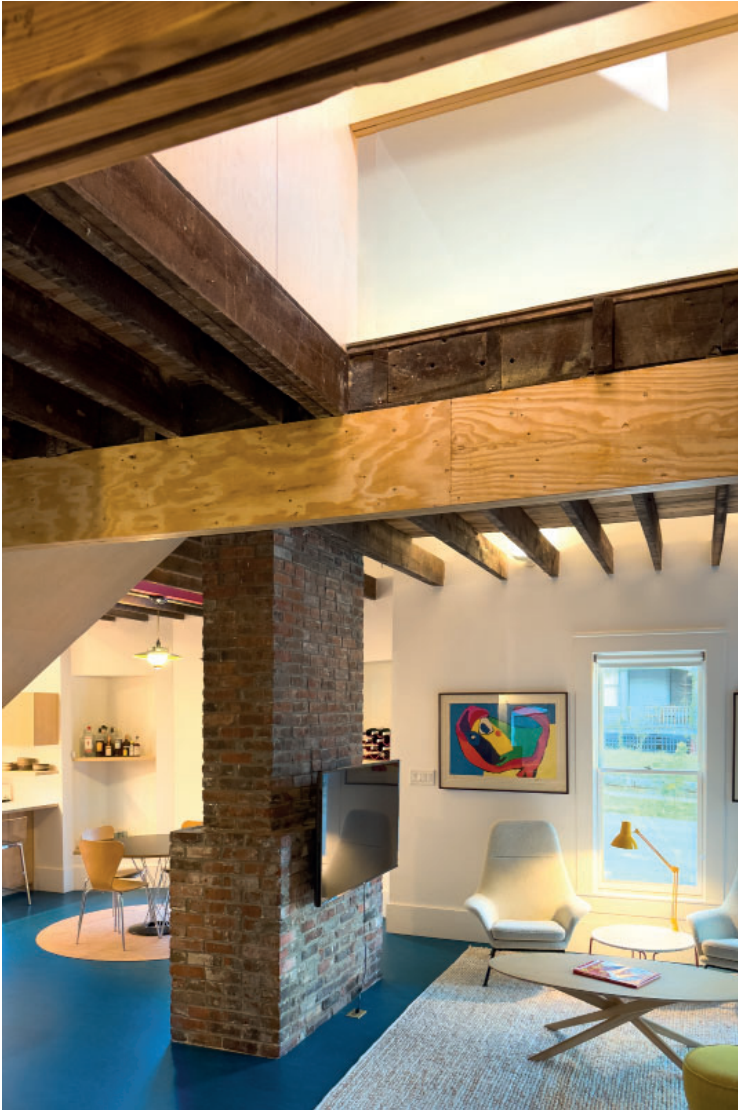
2023 Interior Lower Level. Original, altered, and inserted framing open the floor to the roof at the entry where a skylight accentuates the layers at the entrance hall. Photo by Robert Batey Photography.
