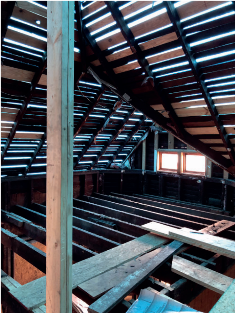
JAN 2021 Extraction during deconstruction. Photo by author.
