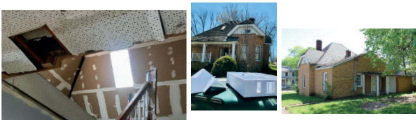
2019 Found condition as encountered by architects.
